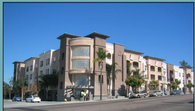
The 90 unit Talmadge Senior Village was partially funded by the City Heights Redevelopment Agency
